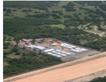
Bechtel, Kitona Training Centre 2700m 2
