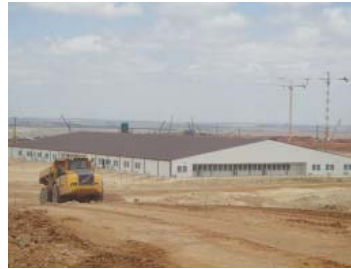
Roshcon Site Services, Kusile Power Station 12000m 2
